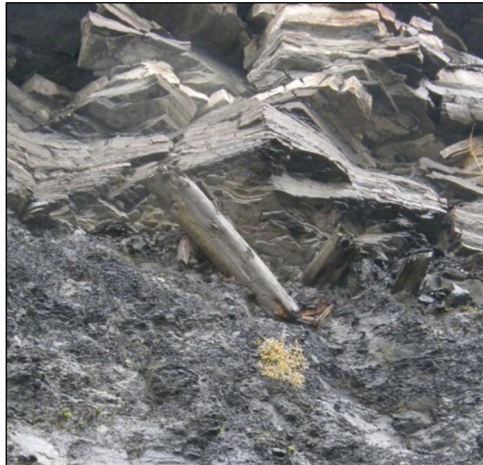
Spireslack_11 P2: Wooden pit prop in situ within the coal workings. The wooden props were used to hold up the roof of the workings as the coal was extracted. The prop, sitting above packed mine waste in the photo, has since collapsed due to the overlying weight of rock (sandstone) above. © BGS, NERC.
